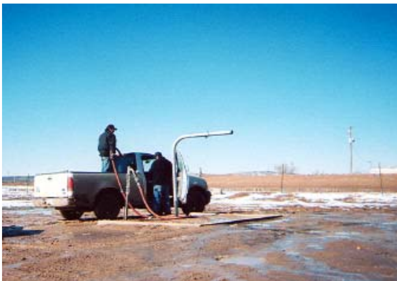
Picture 7. Many residents on the reservations get their water from community wells like this one at the Pinon Community Center, Navajo Nation
