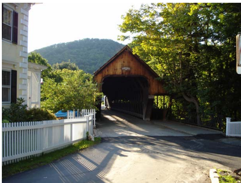
Covered bridge in Woodstock, VT
