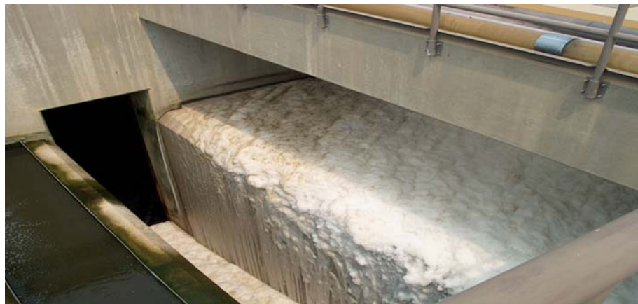
Scum being removed from the secondary treatment
